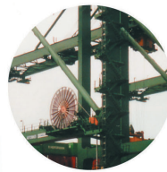
High-stress rubber cables (PNCT-B, PNCT-RF)
