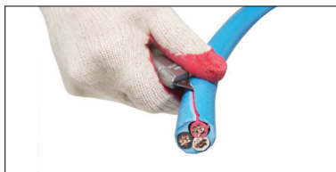
Cut down the sheath from the thinnest point
